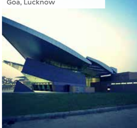
Airports - Bengaluru, Surat, Goa, Lucknow
