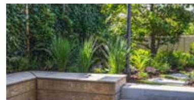
Fixing Stone on wall
