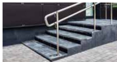
Staircases & Metal Railings
