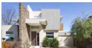
Vertical cladding of Stones
