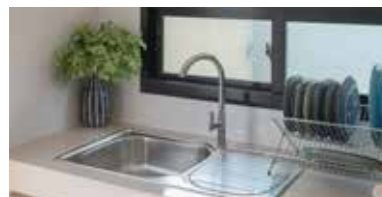
Kitchen Sink Fixing
